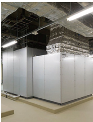
Installation of air conditioning equipment
