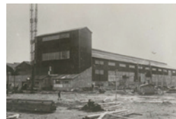
Harima Factory under construction
