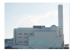
Senboku Clean Center [Primary equipment improvement works] 300 t/day Capacity (150 t/day x 2 incinerators) Power output: 9.300 kW Osaka Prefecture Location
