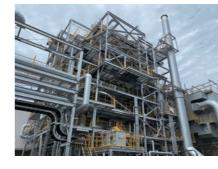
[Biomass power plant] Combustion system: Fuel: Boiler evaporation rate: 25 t/h (maximum) Steam specifications: 5.9 MPaG, 425°C (rating) Power output: Location:
