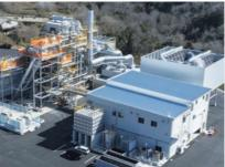
[Biomass power plant] Combustion system: Fuel Boiler evaporation rate: 50 t/h (maximum) Steam specifications: 6.0 MPaG, 425°C (rating) Power output: Location:
