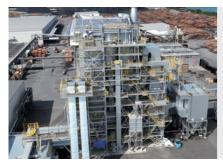
Hyuga Plant, Chugoku Lumber Co., Ltd. [Biomass power plant] Combustion system: Circulating fluidized bed Fuel Wood fuel Boiler evaporation rate: 65 t/h (maximum) Steam specifications: 6.0 MPaG, 460°C (rating) Power output: 14,500 kW \_ocation Miyazaki Prefecture
