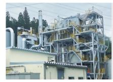
Kumamoto Clean Energy Co. [Biomass power plant] Combustion system: Traveling stoker Fuel: Wood fuel Boiler evaporation rate: 12 t/h maximum) Steam specifications: 4.2 MPaG, 405°C ratina) 1.990 kW Power output: Kumamoto Prefecture \_ocation:
