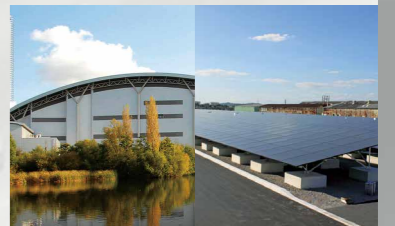
Delivery of an Energy from Waste plant in Europe (2010) Construction of the Takuma Solar Power Plant (2013)
