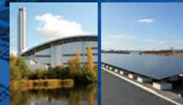
Delivery of an Energy from Waste plant in Europe (2010) Construction of the Takuma Solar Power Plant (2013)
