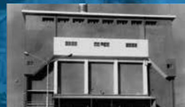
Japan's first 24 hour operating waste incineration plant (1963)
