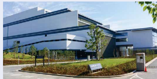
Waste incineration plants
