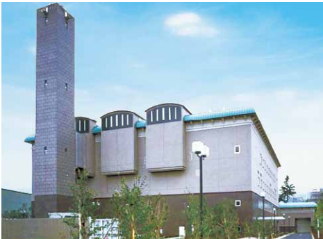
The Inariyama Environmental Center
