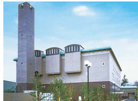
The Inariyama Environmental Center
