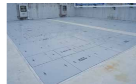
Moving Bed Upflow Continuous Sand Filtration System (high-speed) Treatment capacity: 29,500 m 3 per day
