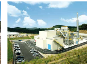
Plant that generates power from industrial waste and provides heat to a plantation
