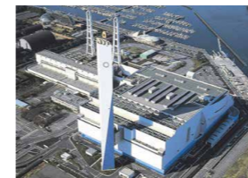
Energy from Waste plant
