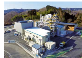
Wood Chip Biomass Power Plant Generating capacity: 1,990 kW
