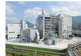
Wood Chip Biomass Power Plant Generating capacity: 22,100 kW
