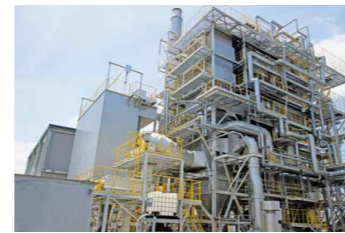
Biomass Power Plant
