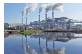
Bagasse-Fired Boiler Plant (Thailand)
