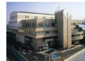
Bulky garbage crushing plant
