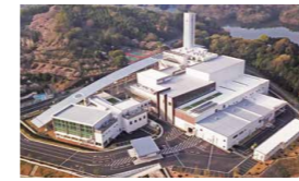
Waste-to-Energy Plant (DBO Project) Treatment capacity: 174 tons per day Generating capacity: 3,800 kW
