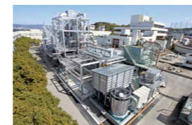
Sludge-Fueled Power System Demonstration Plant Treatment capacity: 35 wet tons per day (with moisture content of about 70%) Generating output: About 100 kWh/h
