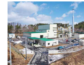
Industrial waste treatment plant
