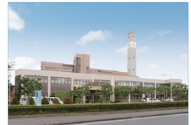
Project name Sakado West Disposal Center Incineration Facility Primary Equipment Improvement Project Capacity Incineration facility: 80 tons per day (40 tons per day × 2 units) Power output: 160 kW Location Saitama Prefecture
