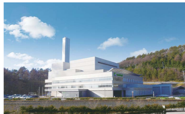
High-efficiency waste-fueled power plant (processing capacity: 110 tons per day) (Delivered in 2016 to the Neighborhood of the Lake Administrative Affairs Association)
