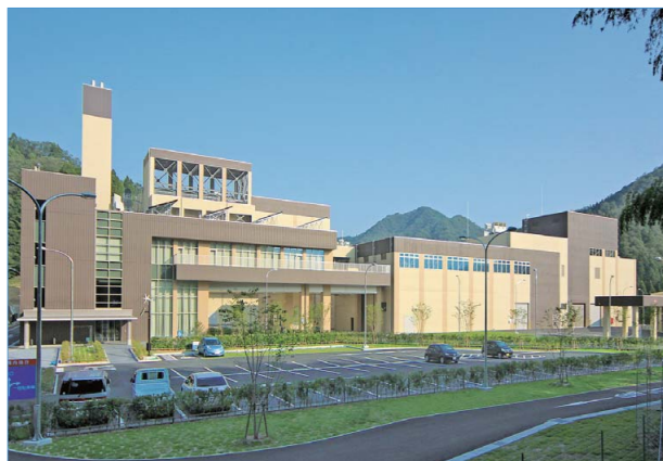
Project name Hokutan Waste Treatment Facility Development and Operation Project Capacity Incineration facility: 142 tons per day (71 tons per day × 2 units) Power output: 2,850 kW Location Hyogo Prefecture
