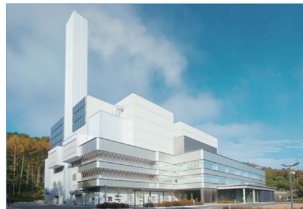
Project name Lakeside District Waste Treatment Facility Development Project Capacity Incineration facility: 110 tons per day (55 tons per day × 2 units) Power output: 2,050 kW Location Nagano Prefecture
