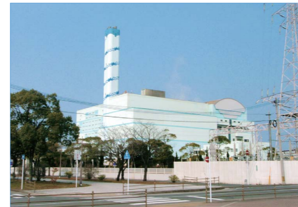
Project name Kogasaki Plant Incineration Facility Improvement Project Capacity Incineration facility: 810 tons per day (270 tons per day × 3 units) Power output: 17,200 kW Location Fukuoka Prefecture
