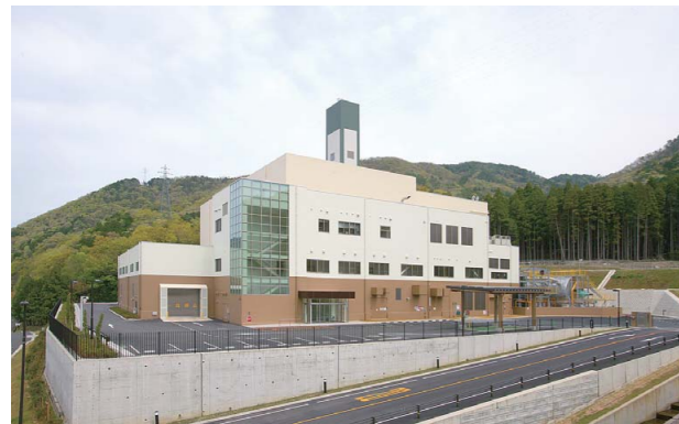
Combined facility comprised of waste incineration and biogas recovery plants (Delivered in 2013 to Nantan Regional Administrative Association)
