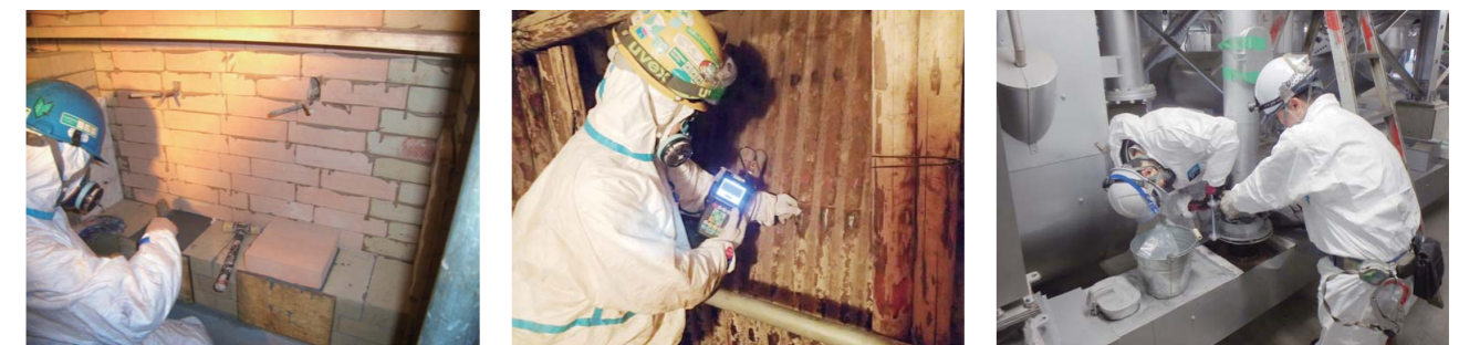
Repairing an incinerator's refractory
