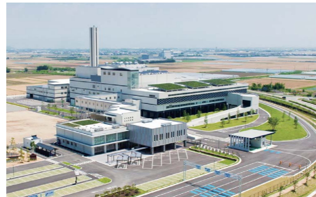
High-efficiency waste-fueled power plant (processing capacity: 163 tons per day) (Delivered in 2016 to Kurume City)
