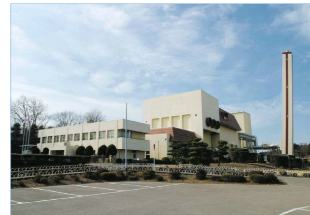
Project name Konan Clean Center Core Equipment Improvement Project Capacity Incineration facility: 100 tons per day (50 tons per day × 2 units) Location Saitama Prefecture
