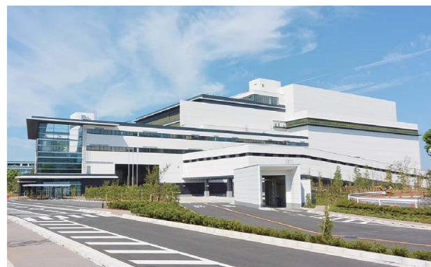
High-efficiency waste-fueled power plant (processing capacity: 600 tons per day) (Delivered in 2014 to the Clean Authority of Tokyo)
