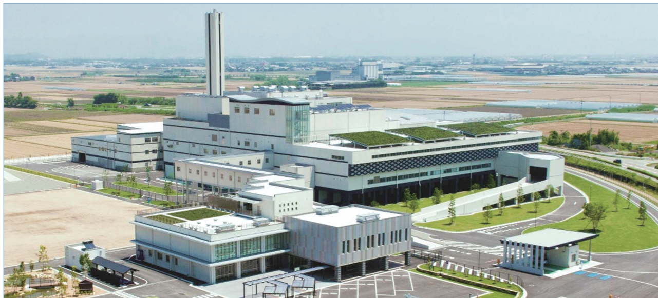
Project name Northern Kurume Solid Municipal Waste Treatment Facility Development and Operation Project Capacity Incineration facility: 163 tons per day (81.5 tons per day × 2 units) Power output: 3,560 kW Location Fukuoka Prefecture
