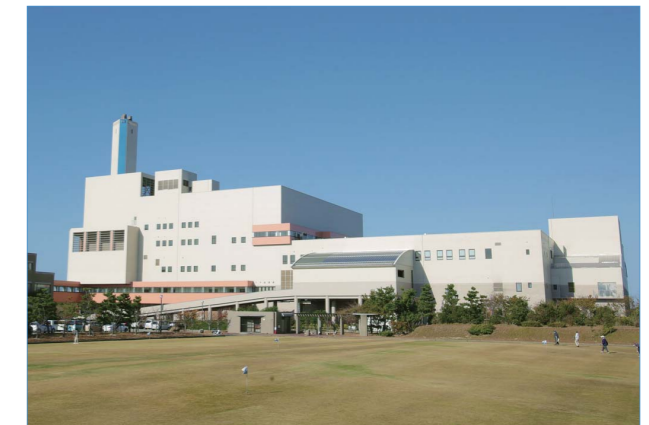
Project name Mattoishikawa Environmental Clean Center Primary Equipment Improvement Project (Plant Construction) Capacity Incineration facility: 240 tons per day (80 tons per day × 3 units) Power output: 2,900 kW Location Ishikawa Prefecture
