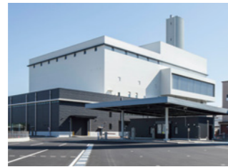
Waste incineration plant
