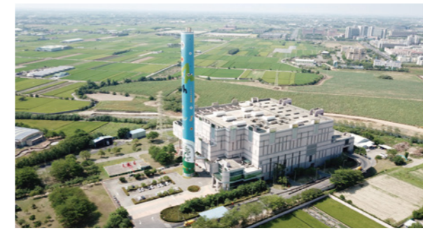
Energy from Waste plant
