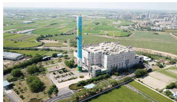
LuTsao Incineration Plant, ChaiYi County (Taiwan)
