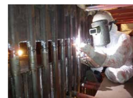
Replacing boiler tubes
