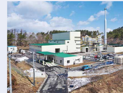
Industrial waste treatment plant
