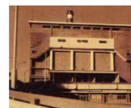
(6) Japan's first 24 hour operating waste incineration plant
