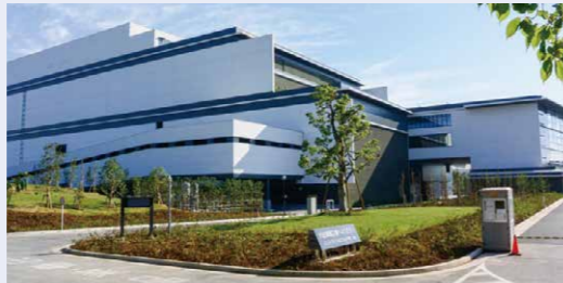
Waste incineration plants
