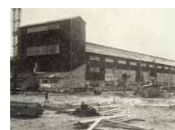
(2) Harima Factory under construction
