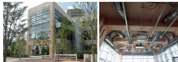
Hospital (Adachi-ku, Tokyo)
