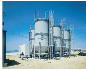
Upflow moving-bed filtration system
