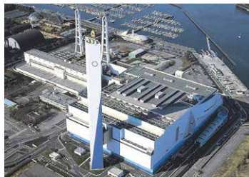
Energy from Waste plant
