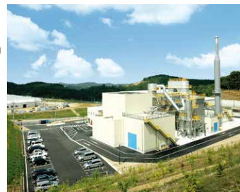
Plant that generates power from industrial waste and provides heat to a plantation
