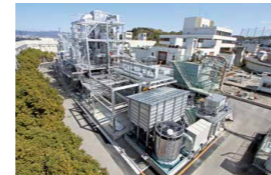
Sludge-Fueled Power System Demonstration Plant Treatment capacity: 35 wet tons per day (with moisture content of about 70%) Generating output: About 100 kWh/h
