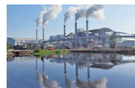
Bagasse-Fired Boiler Plant (Thailand)
