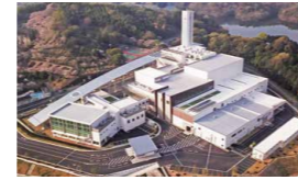
Waste-to-Energy Plant (DBO Project) Treatment capacity: 174 tons per day Generating capacity: 3,800 kW
