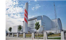
Waste-to-Energy Plant (China) Treatment capacity: 1,600 tons per day Generating capacity: 30,000 kW
