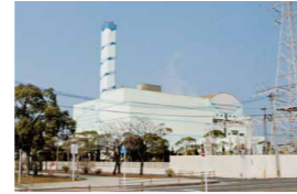
Waste-to-Energy Plant (Primary equipment improvement project) Treatment capacity: 810 tons per day Generating capacity: 17,200 kW
