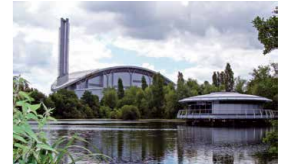
Waste-to-Energy Plant (UK) Treatment capacity: 1,370 tons per day Generating capacity: 36,650 kW
