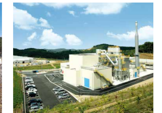
Plant that generates power from industrial waste and provides heat to a plantation
