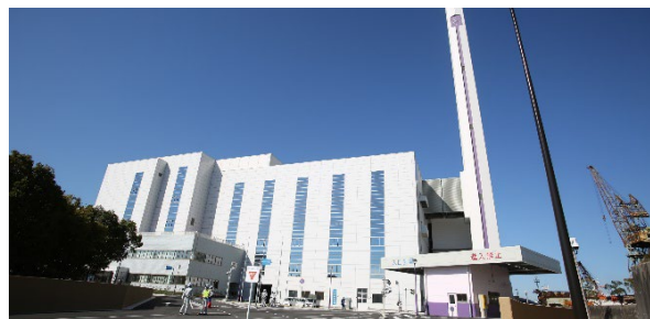
Municipal solid waste treatment plants
