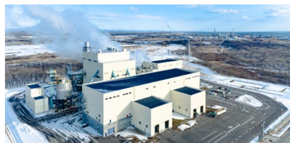
Biomass power plants
