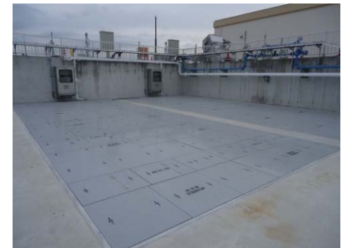
Moving bed upflow continuous sand filtration system (high-speed) Treatment capacity: 29,500 m 3 /day
