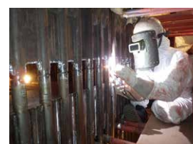
Replacing boiler tubes
