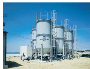
Upflow moving-bed filtration system
