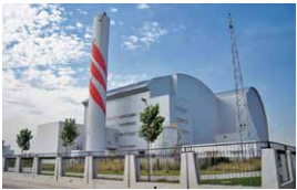
Waste-to-Energy Plant (China) Treatment capacity: 1,600 tons per day Generating capacity: 30,000 kW
