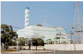
Waste-to-Energy Plant (Primary equipment improvement project) Treatment capacity: 810 tons per day Generating capacity: 17,200 kW
