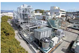
Sludge-Fueled Power System Demonstration Plant Treatment capacity: 35 wet tons per day (with moisture content of about 70%) Generating output: About 100 kWh/h
