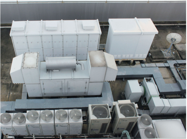
Emergency rooftop generator for providing emergency power*
