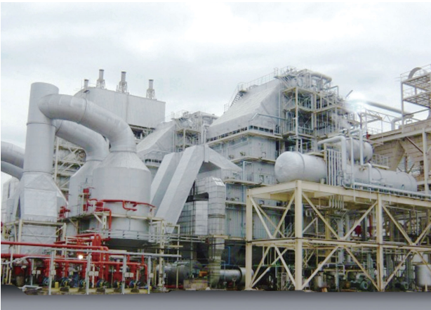
Bagasse-fired boiler installation example
