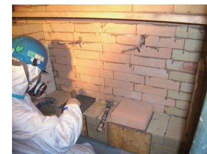
Repairing an incinerator's refractory
