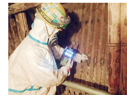
Measuring the thickness of boiler water tubes
