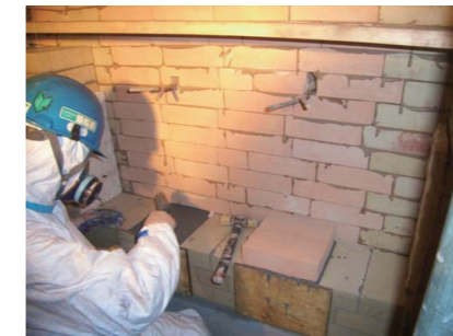
Repairing an incinerator's refractory
