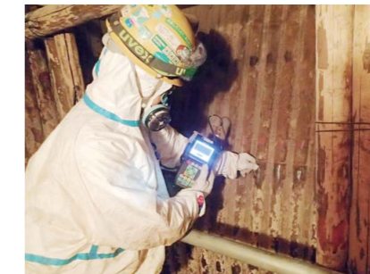
Measuring the thickness of boiler water tubes
