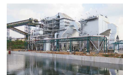
Bagasse Fired Boiler Plant (Thailand)
