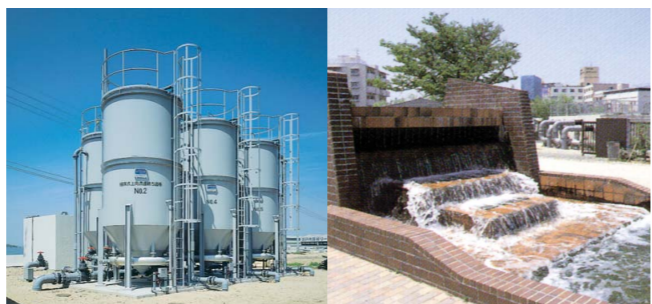
Continuous up-flow sand filter Purification of park pond water
