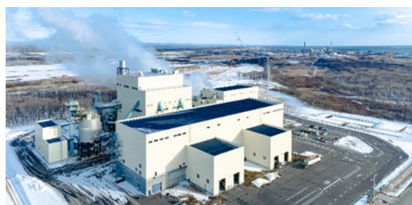
Biomass power plants
