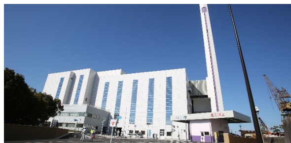
Municipal solid waste treatment plants
