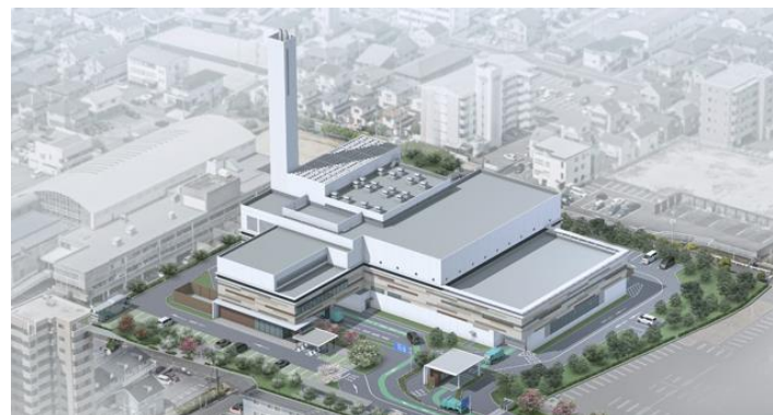
Okayama City: completion image
