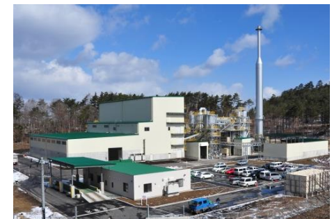
Industrial waste treatment plants
