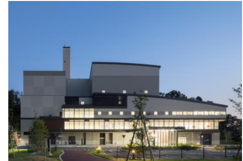
Waste incineration plants
