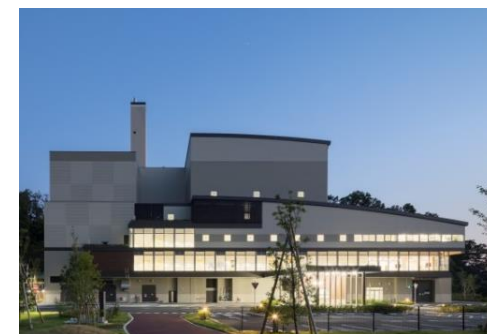
Waste incineration plants
