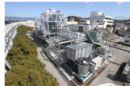
Sludge-Fueled Power System Demonstration Plant
