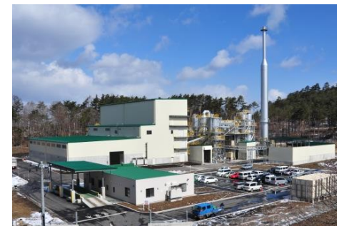
Industrial waste treatment plants
