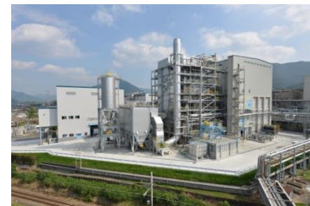
Biomass Power Plant
