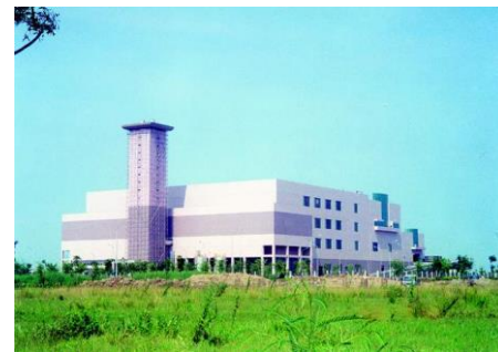
Waste-to-Energy Plant (Taiwan)
