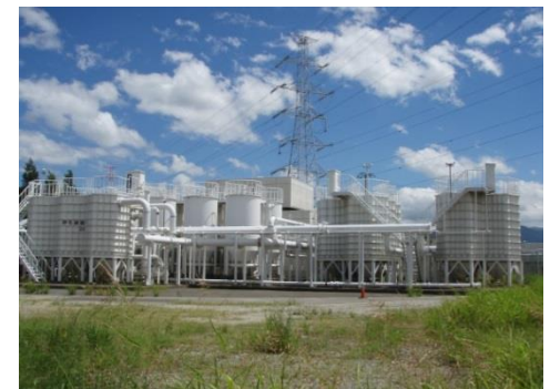
Moving-bed sand filtration systems
