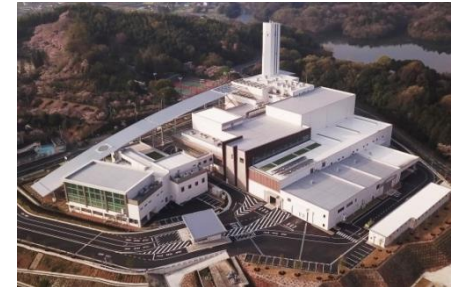
Waste-to-Energy Plant DBO Project
