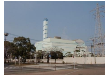
Waste-to-Energy Plant Primary equipment improvement project
