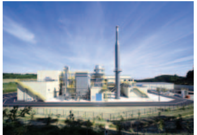
Industrial Waste Treatment Plant with Power Generator
