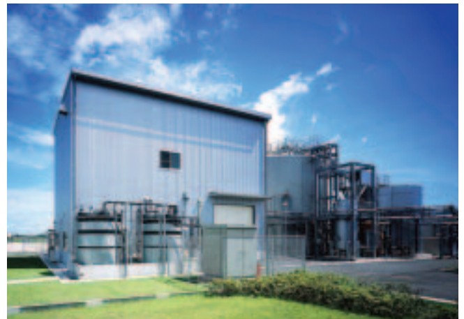
Demonstration plant showcasing a system for recovering energy from distilled spirit lees (see page 15)
