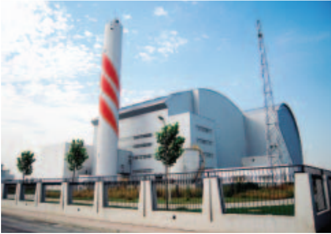
Beijing Gaoantun Waste-to-Energy Plant (CHINA)
