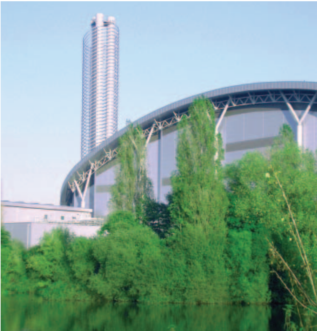
Lakeside Energy from Waste Plant (U.K.)
