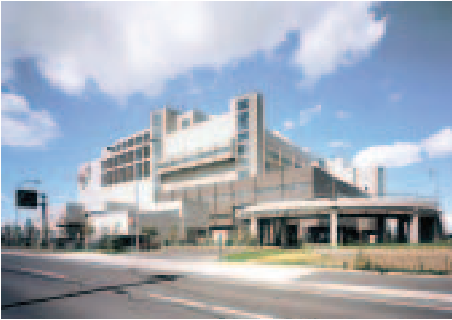
Shiroishi Incineration Plant (Sapporo, JAPAN)
