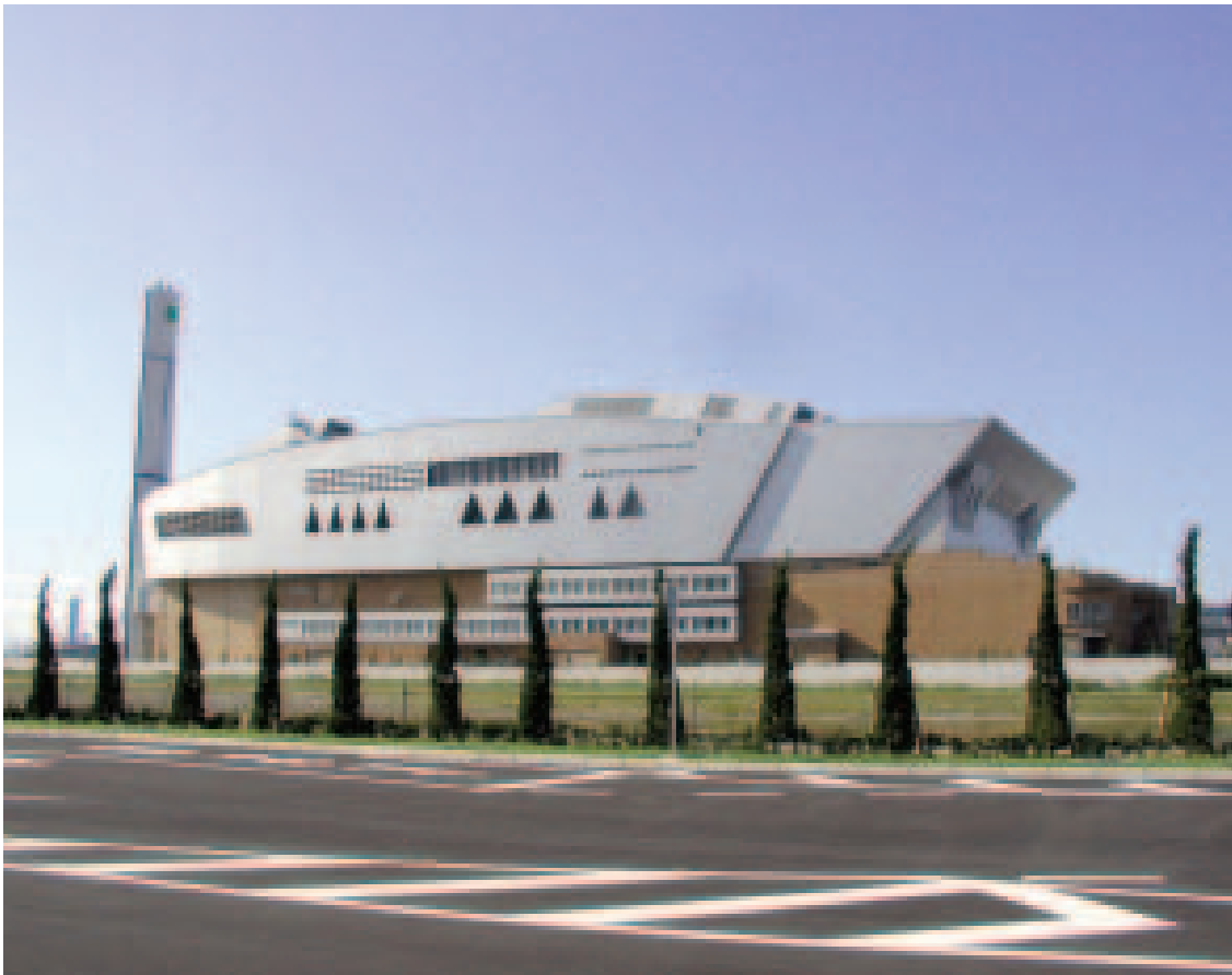
Amagasaki Clean Center (Amagasaki, JAPAN)
