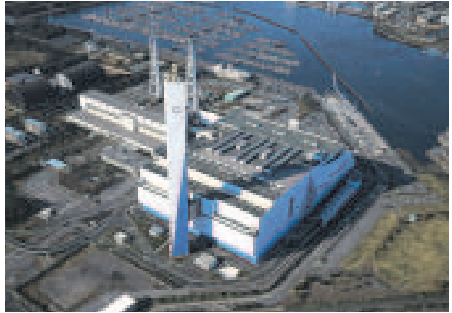
Shin-koto Incineration Plant (Tokyo, JAPAN)
