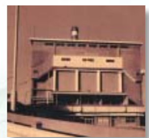
Japan's first waste incineration plant
