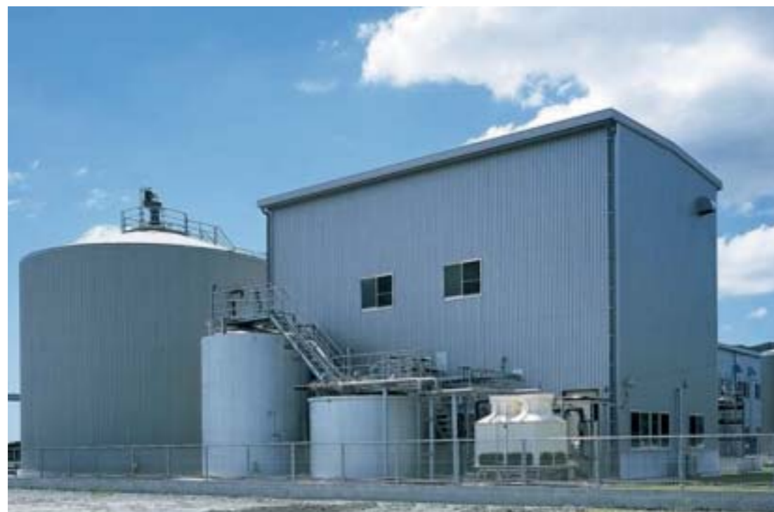
Demonstration Plant for Hydrogen and Methane of Shochu Lees
