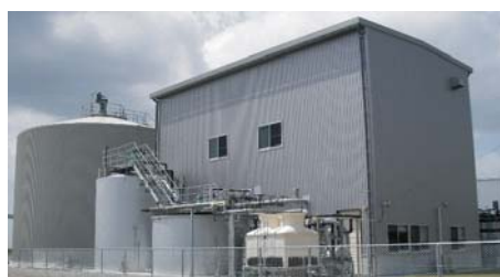
Demonstration plant for energy recovery from SHOCHU residue by alkaline pretreatment-hydrogen-methane fermentation
